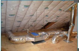
A slim duct unit was installed above the great room in the attic. It provides the concealed look of central air with the efficiency of a mini-split!
