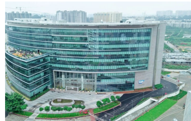
Office building of ABS customer
