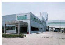
FUJITSU GENERAL (SHANGHAI) CO., LTD. Technical Center
