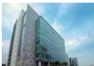
ABS Aircon Engineers Private Ltd. (India)
