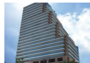
Fujitsu General (Thailand) Co.,Ltd. Bangkok Office (Thailand)
