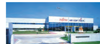
Fujitsu General (Thailand) Co., Ltd. (Thailand)
