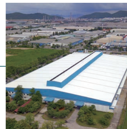
Fujitsu General (Thailand) Co., Ltd. (Thailand) Factory-2
