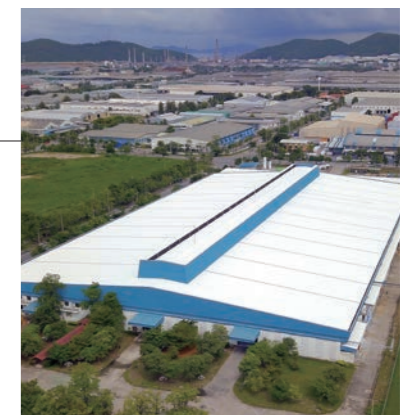
Fujitsu General (Thailand) Co., Ltd. (Thailand) Factory-2
