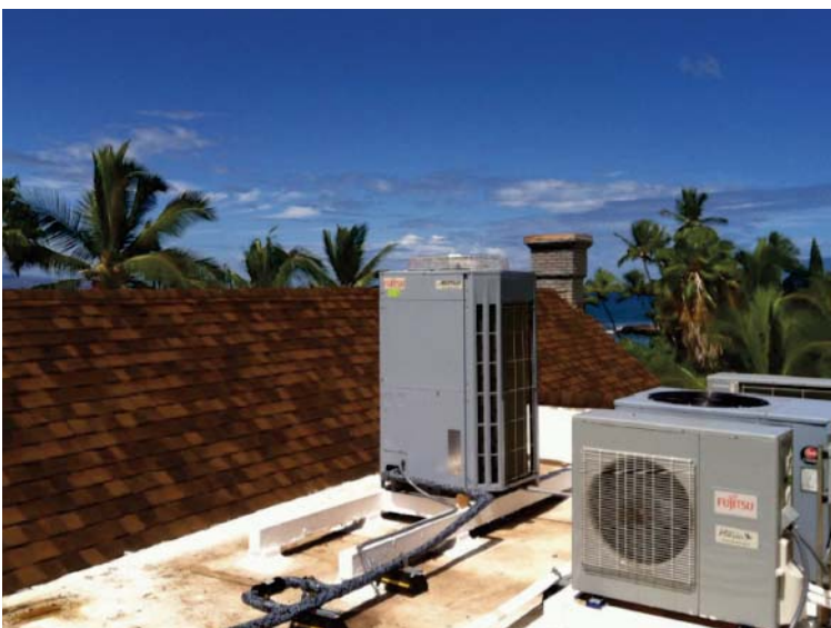
The units were coated for salt water protection. That included the sheet metal, giving it a grey color.
