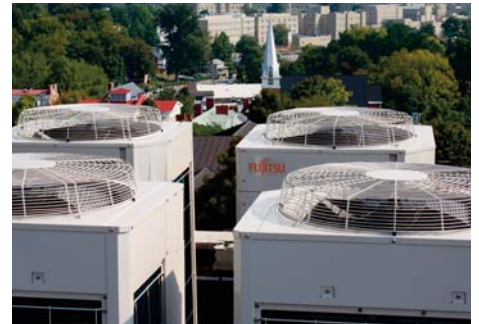
The outdoor units were installed on the upper roof and on various lower roofs. Mostly 6-ton outdoor units were used.
