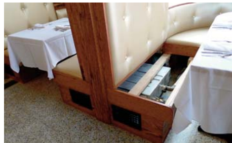
Slim duct units are installed underneath bench seating in the restaurant.
