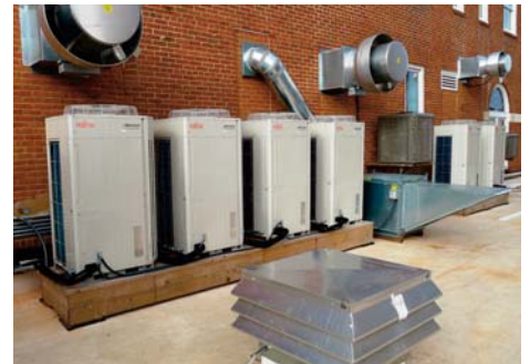
The outdoor units were installed on the upper roof and on various lower roofs. Mostly 6-ton outdoor units were used.
