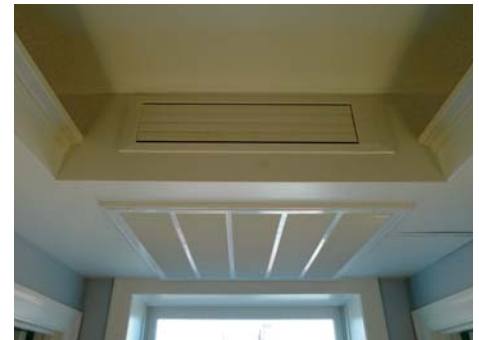
Guest room corridors are served by a slim duct unit at both ends. They are installed with an Auto Louver Grille Kit and a large filter grill to provide filtration and service access.
