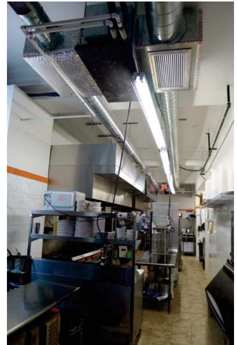
The kitchen is served by two high static ducted units and significant quantities of makeup air.
