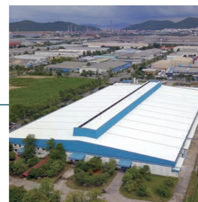
Fujitsu General (Thailand) Co., Ltd. (Thailand) Factory-2
