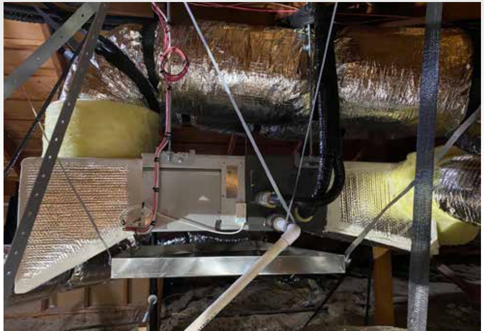
Medium Static Pressure Duct Indoor Unit.
